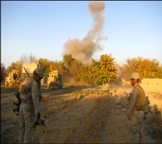
EOD taking down a wall
