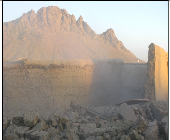
A house before demo
